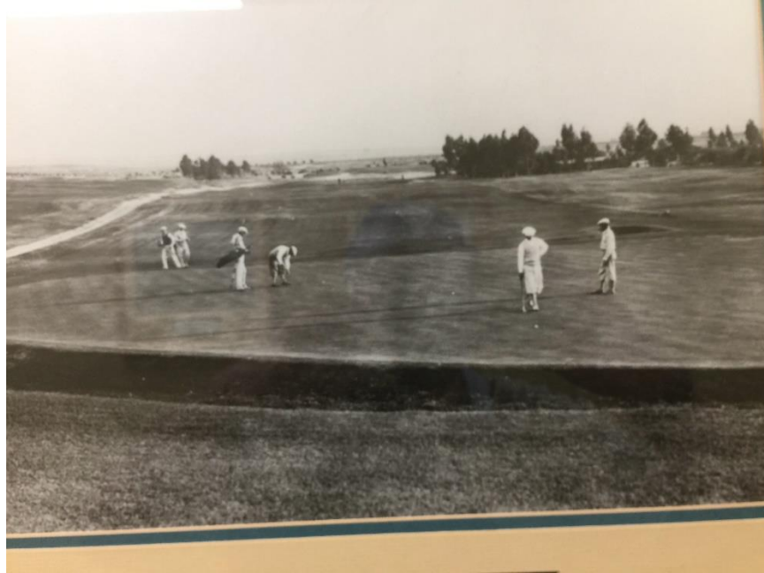
Example of Watson's early trench bunkering over the back of the green compliments of San Diego Country Club
