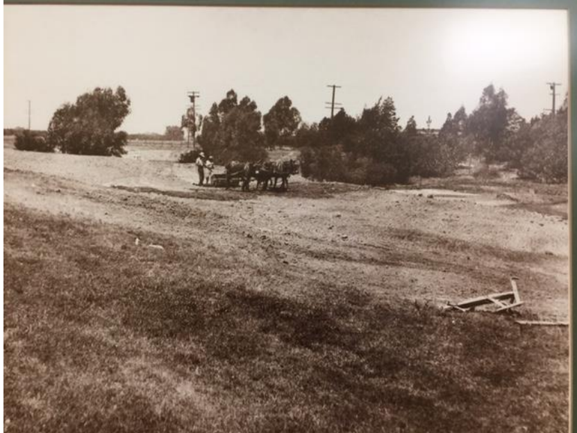
Watson's Construction crew in action, compliments of San Diego Country Club
